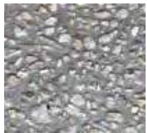
Richmond Exposed Aggregate Driveway
